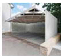
© J.L. Deru - Daylight
